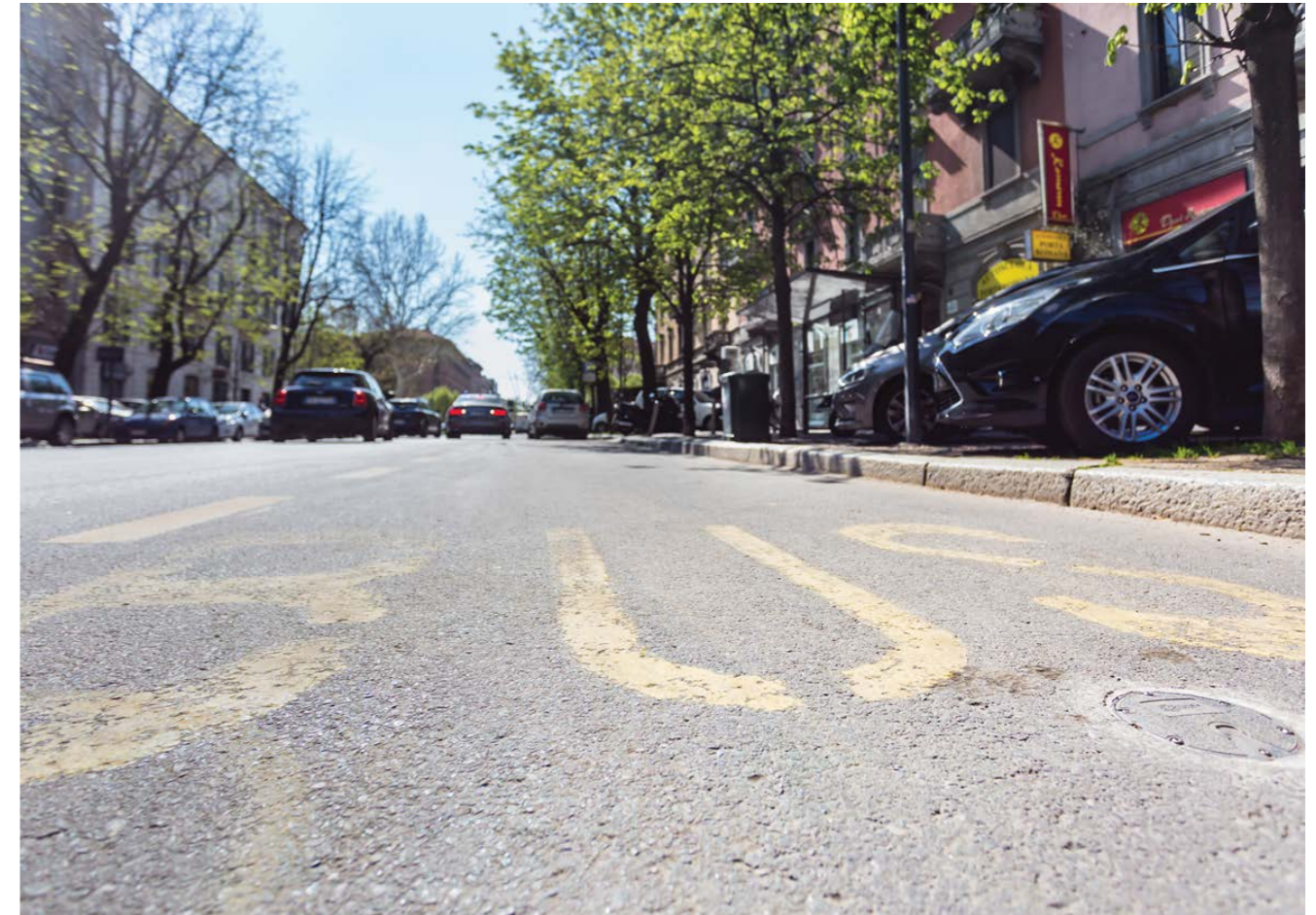
SMART PARKING SENSOR – BUS STOP VIA LAZZARO PAPI
